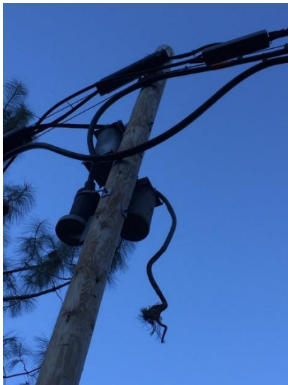
Retired Copper Cable Infrastructure
