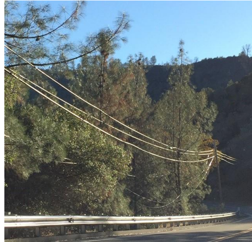
Low Hanging Cable and Tree Limb Overhang
